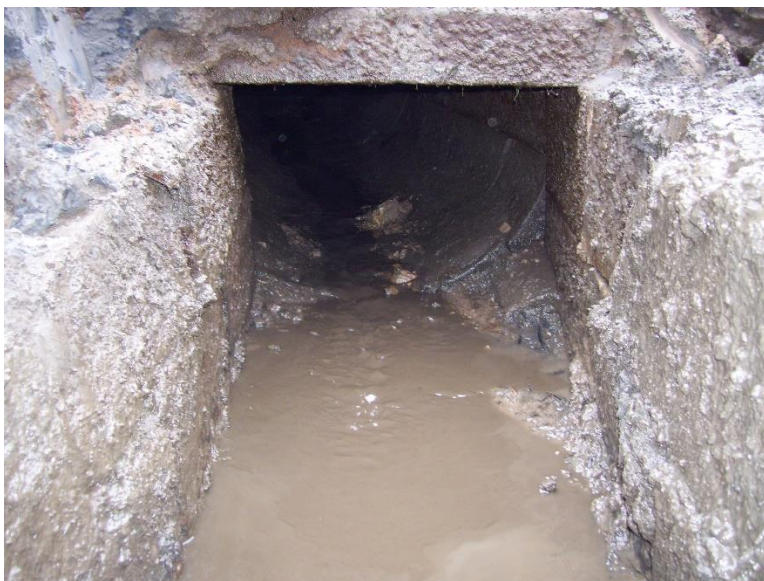
Photo F – Exposed outlet end of 900mm CRT culvert
